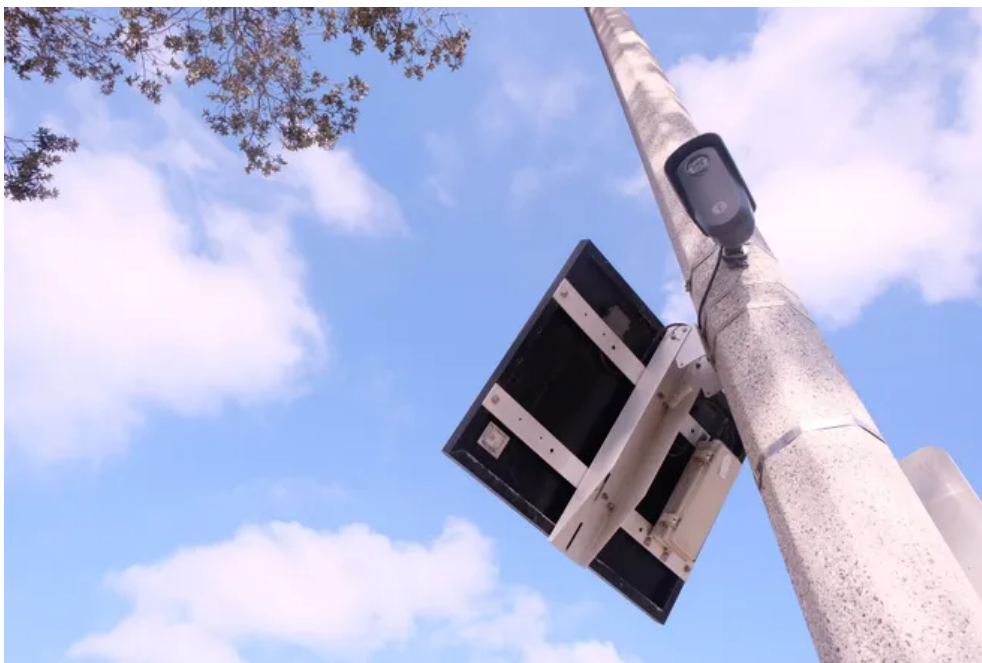
A Flock Safety-branded license plate reader camera site on a lamppost in Ventura, California, on Sept. 9, 2025. ISAIAH MURTAUGH/THE STAR
